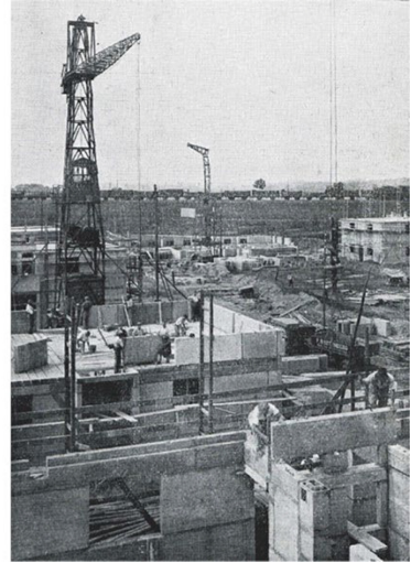
Fig. 6. Left: posters of the “Eliobeton-Pinottini” system and the “Galpomice” company; respective source: AA. VV., Atti e Rassegna Tecnica. Society of Engineers and Architects in Turin, Turin, 1954 | Pagliuca A. Materials Made in Italy, Avanguardia Italiana nell’Industria delle Costruzioni del Primo ‘900”, Gangemi Editore, Rome, 2019; Right: construction site of a building made of pumice stone concrete slabs - source: Griffini E., Costruzione Razionale della Casa, Hoepli, Milan, 1932.
