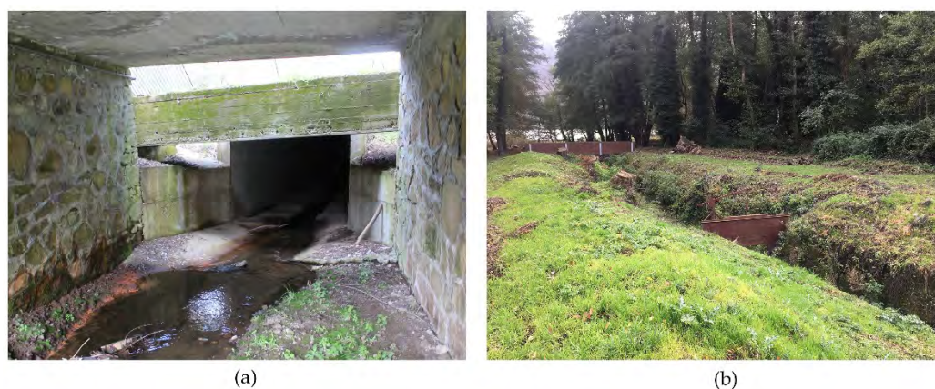
Figure 11. Constructions along the Torrente Laghi channel.
