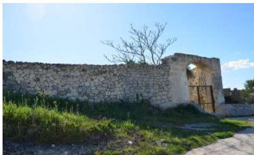
Fig.6,7 – construction of dry stone “paretoni” at Cava del Sole Matera. Source: Giuseppe Andrisani Archive.
