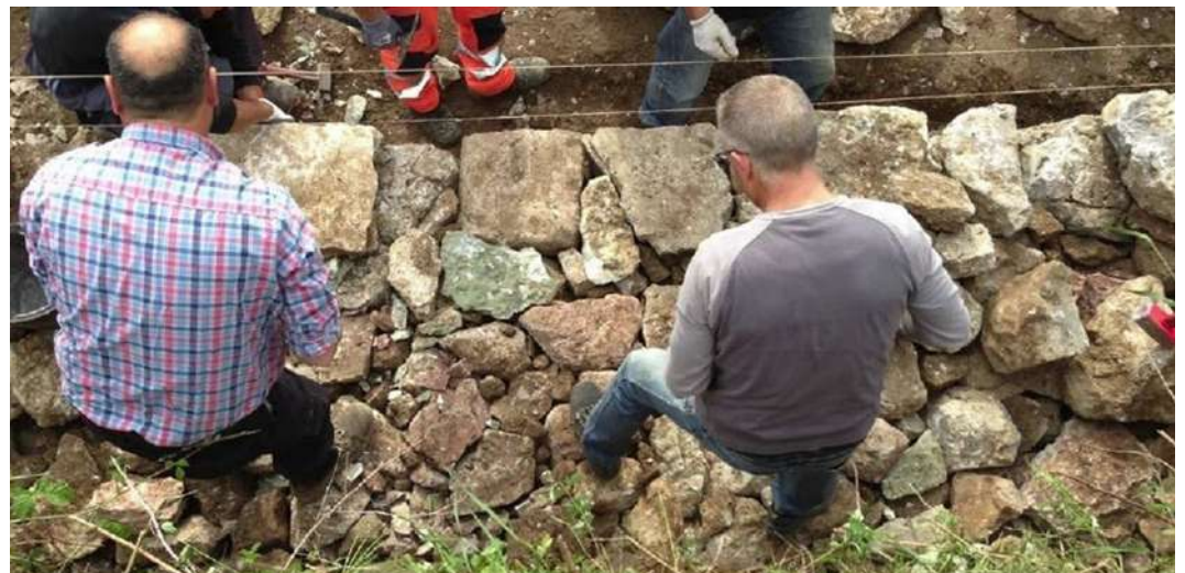
Fig.5 – construction of dry stone walls in the Park of the Rupestrian Churches of Matera. Source: Giuseppe Andrisani Archive.
