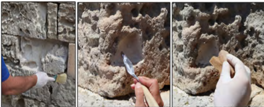
Figure 13. Filling of the alveolized cavity of the sample ashlar on the left side of the facade of San Francesco d'Assisi with an experimental mortar containing aerial lime and an acrylic-urethan product in aqueous solvent developed by the industrial partner Icap Leather ChemSpA.
