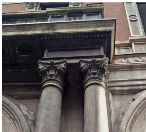
Figure 1. Example of black crust formation.
