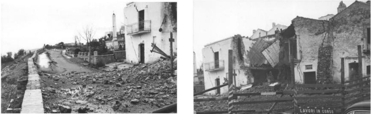
Figure II.16 - Effects of CS landslide reactivation in Craco in January 1965
