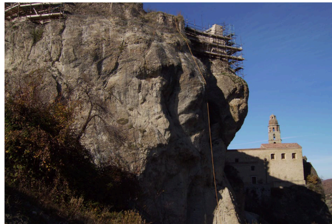
Figure 10. Consolidation work on the conglomerates and the buildings.
