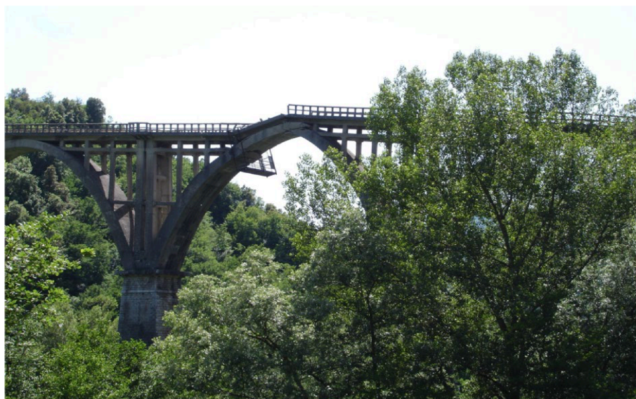
Figure 14. View of the Calabro-Lucane railway bridge in Lagonegro.
