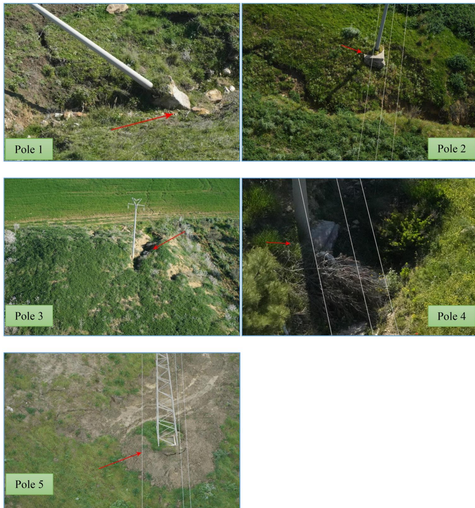
Figure 2. Aerial photos of electrical poles identified as test-cases. Date of acquisition: pole (1) 2/18/2023, pole (2) 3/22/2023, pole (3) 2/14/2023, pole (4) 4/19/2023, and pole (5) 2/13/2023.
