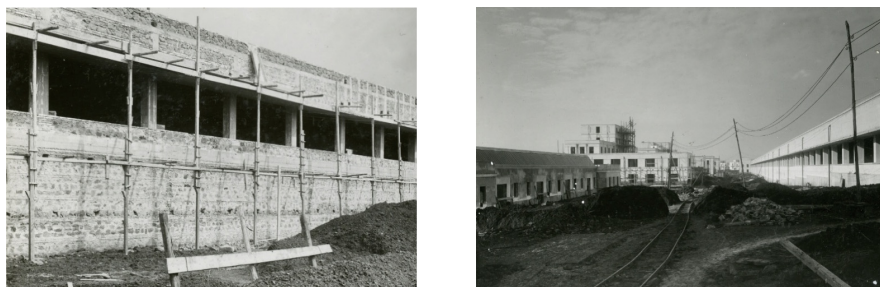
Fig. 8. On the left, external photo of the hydrodynamic tank under construction, with scaffolding. On the right, external view of the construction site of the Guidonia Higher Studies Directorate of Experiences in the construction phases: detail of the track for the transport of construction site equipment and goods (fonte: Archivio Centrale dello Stato- Fondo - Archivio degli organi politici e amministrativi dello Stato, fondo- direzione generale del demanio, subfondo - divisione demanio, serie - costruzione aeroporti, fotografie).
