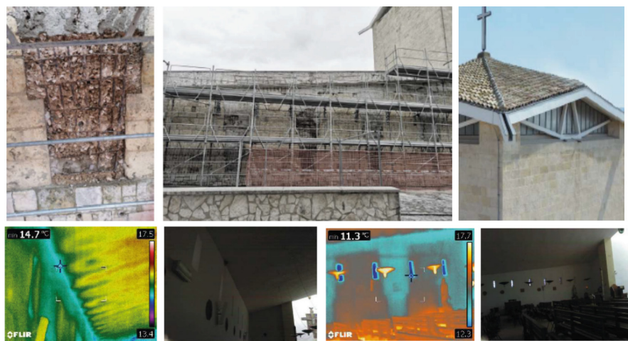
Fig. 7. Above, from left to right: detail of reinforced concrete pillar, interventions carried out on the facades (2018), bell tower (2024); below, from left to right: thermographic surveys – hall floor, hall masonry (photos by the authors).
