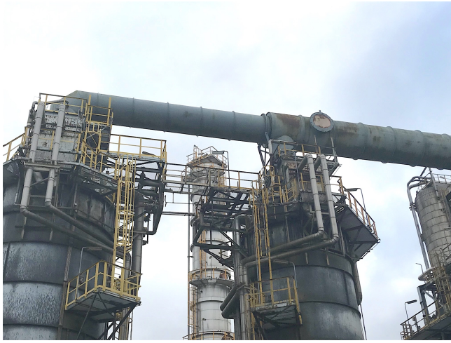
Fig. 2. Oil and Gas refinery in Germany.
